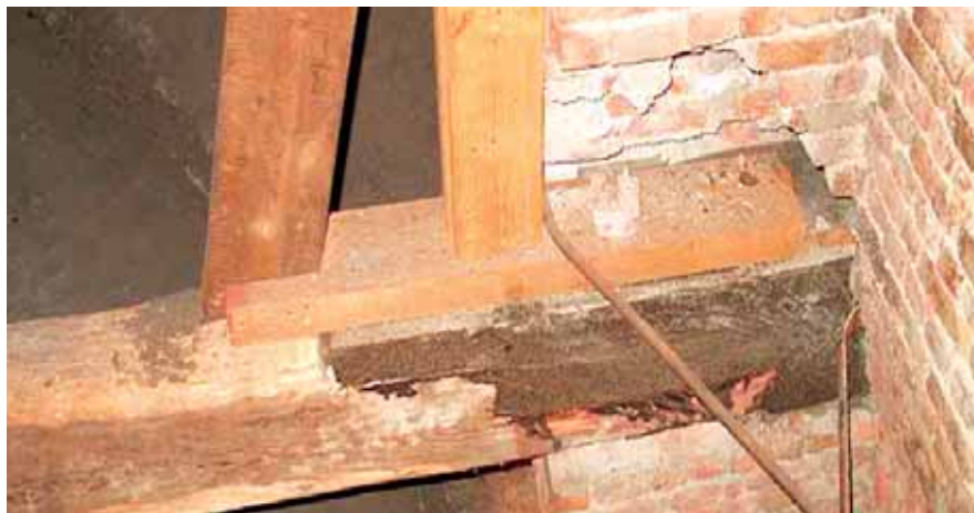
Epoxyherstelling.
